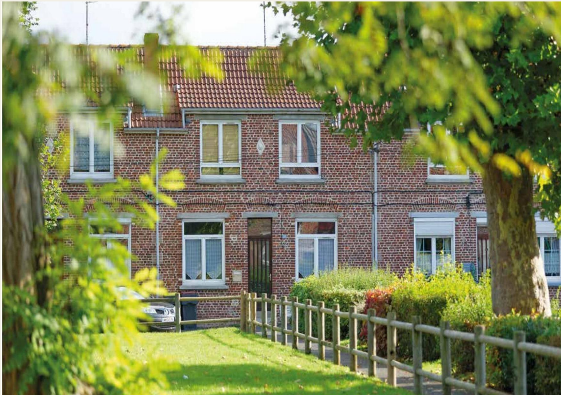
Cité Barrois, Pecquencourt — mining-era brick housing under renovation
